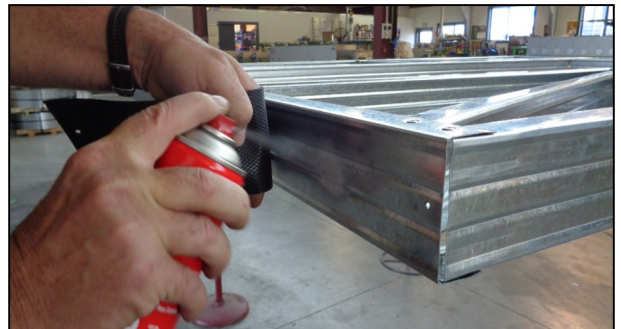
Gluing DPC to the Bottom Plate
