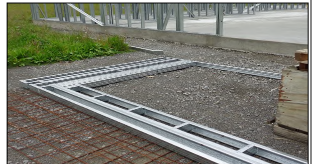
Lay frames around the foundation prior to standing walls
